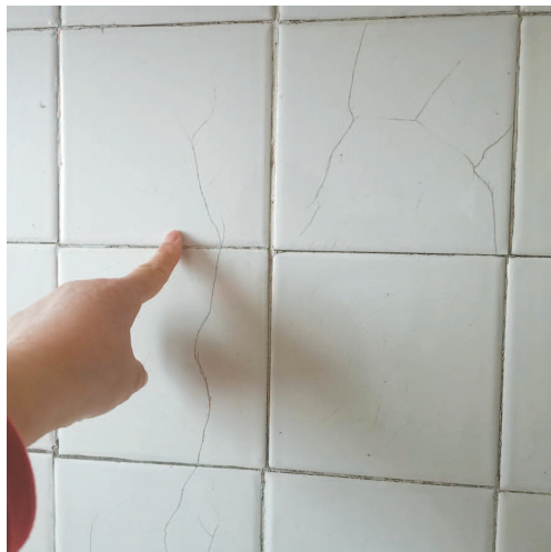
墙壁布满裂缝
